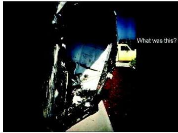
UCI refrigerator which exploded when chemicals were stored in a unit which was not designed for flammables
